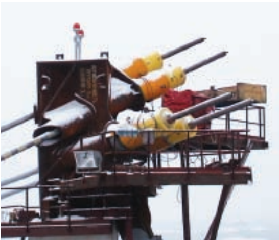
Stylite Internal/External Thread Cylindrical Socket used to anchor roof catenary strand
