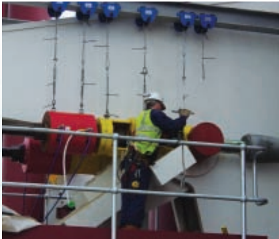
Stylite Conical Socket used to anchor roof support strand.
