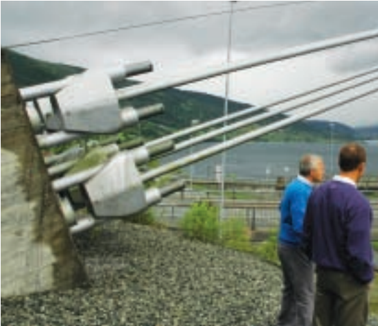
Stylite Block Socket used as main cable anchor
