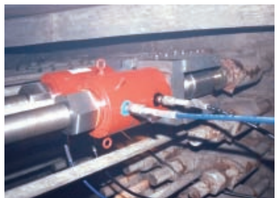
Detensioning of suspension bridge main cable
