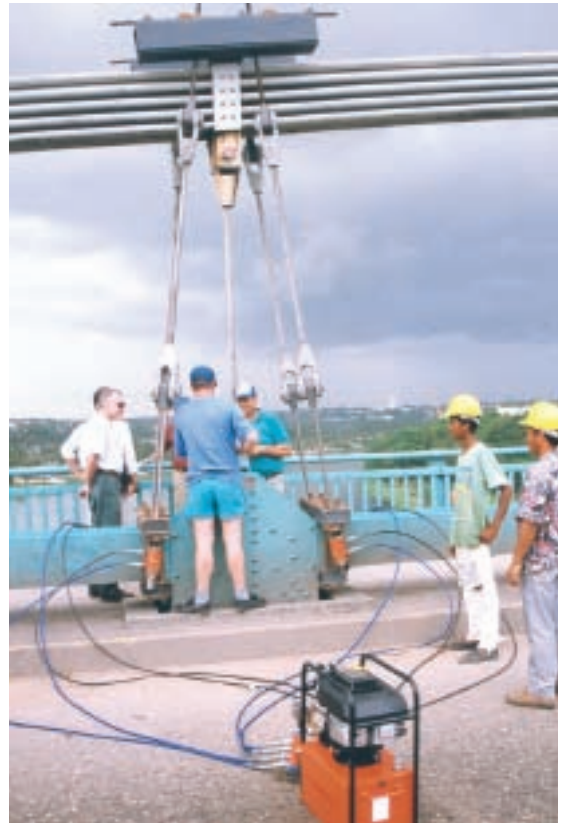
Replacement of hanger cable on suspension bridge
