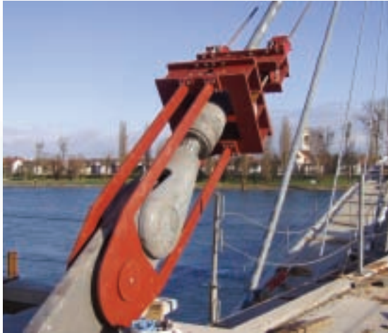
Stylite Adjustable Fork Socket used as deck anchor
