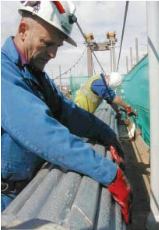
Main Cable inspection on Tamar Bridge, UK
