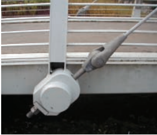
Stylite Fork Socket Adaptor Bar used as deck anchor
